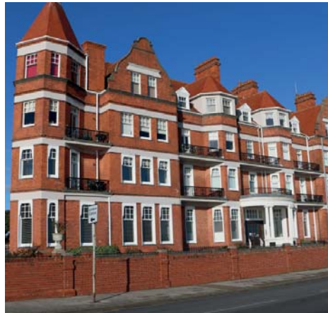
Figure 34 Colchester Institute (Grade II Listed)
