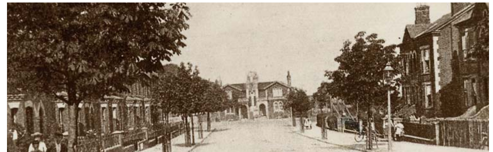
Figure 44 Trees along Station Road, 1910
