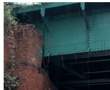
Figure 22 A detail of the railway bridge
