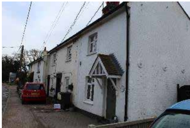
Figure 41 1 and 2 Ivy Cottages
