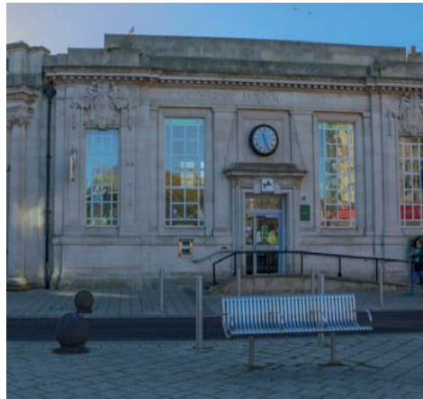
Figure 24 Lloyds Bank Building
