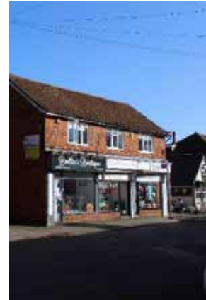
Figure 75 Modern Shop Front
