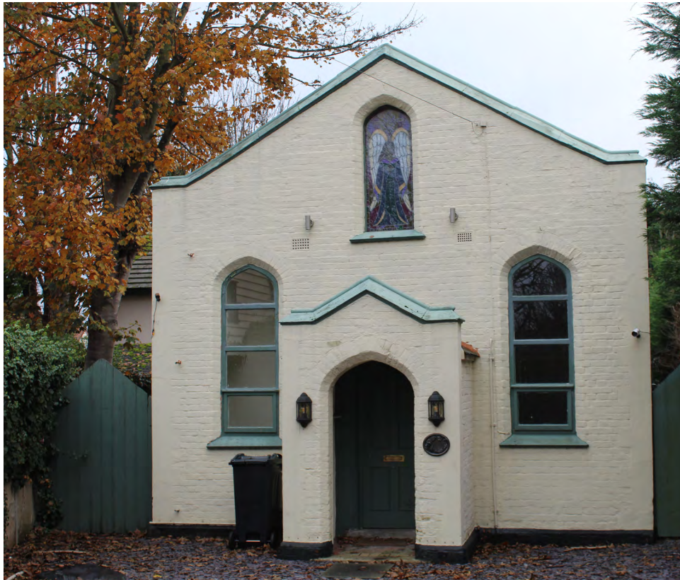
Figure 31 The Old Chapel 30 Colchester Road
