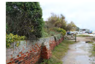
Figure 60 Example of historic walls
