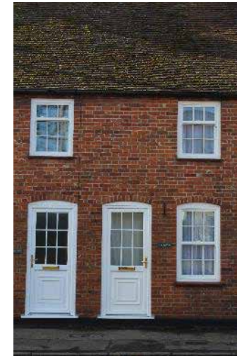
Figure 76 Loss of Architectural Details
