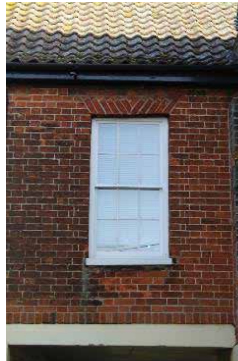
Figure 64 Examples of 'V' shaped red brick lintels
