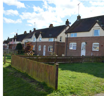
Figure 39 Twentieth century semi-detached houses
