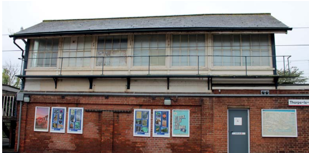
Figure 20 The signal box on Thrope-le-Soken's island platform
