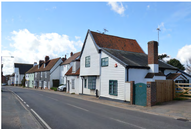
Figure 61 Numbers 45-49 Mill Street
