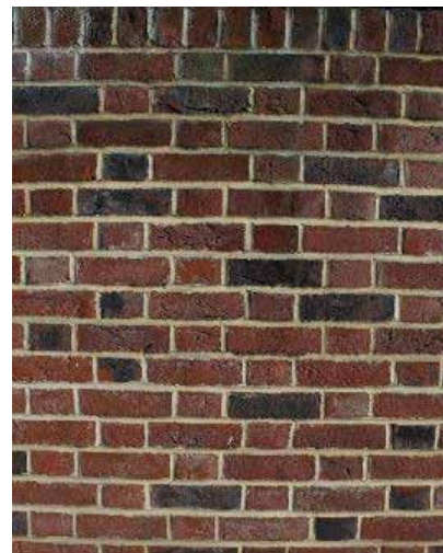
Figure 49 Flemish bond brick-built boundaries contribute to the character of the Conservation Area
