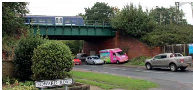
Figure 21 Thorpe-le-Soken railway bridge
